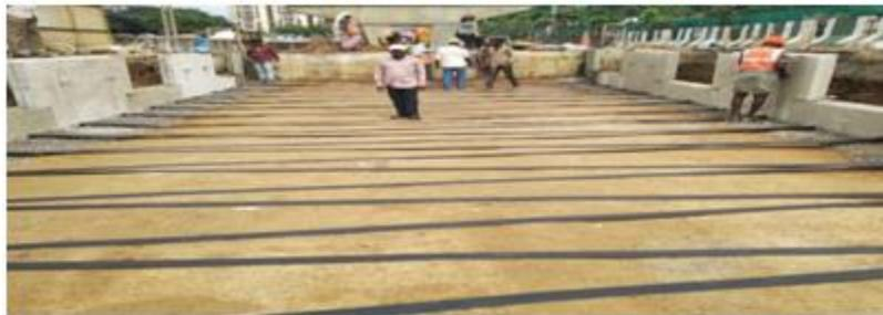
Fig.2: Shows Geo-textile Used in Road Work at Madhapur
