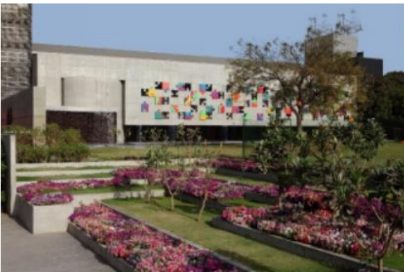
Figure 1: Front facade of Nirma Vidyavihar
