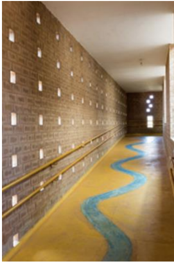
Figure 3: Ventilated Jali corridors
