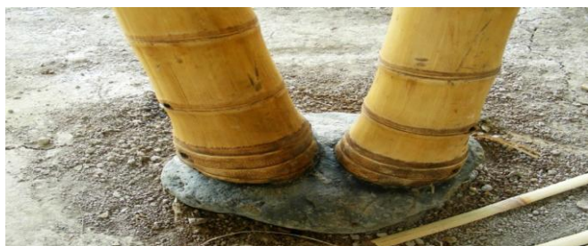
Fig. 3.4 This image indicate the bamboo connected by using a single base connection
