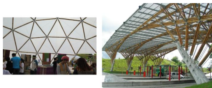
Fig. 3.3 This image indicate the space structure constructed by using bamboo
