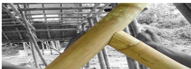
Fig. 3.5 This image indicate the bamboo connected by T-joint
