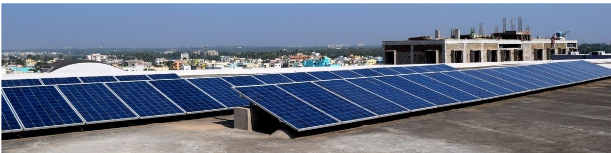
Figure 3. Setup of roof top based 11.2 kW PV system at SOA
