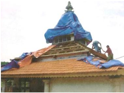
FIGURE 3: Installation of “Marseille” roof tiles on the second and third roof tier (Source: PERZIM)
