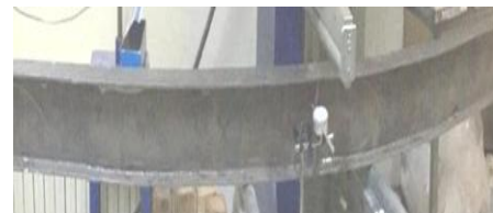
Fig.17: The failure mode for beam with no stiffeners
