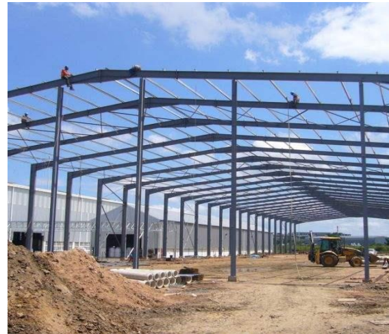
Figure 2. Overall design and building stock of prefabricated buildings.
